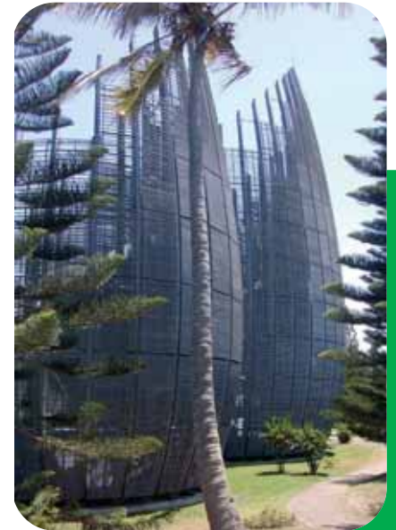
Centre culturel J.M. Tjibaou, structure made of iroko (New Caledonia). © J. Gérard, CIRAD
